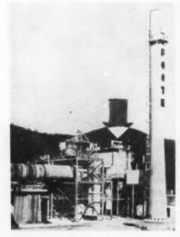
ROTARY KILNS, Buell electrostatic precipitator (arrow), and exhaust stack. Clinker dust is returned to process after separation from kiln exhaust gas. Dust recovery is 97.5 percent efficient-54 tons per day.
